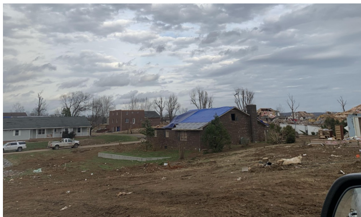
From my aunt's neighborhood. On the left are homes barely touched; on the right is just devastation.
